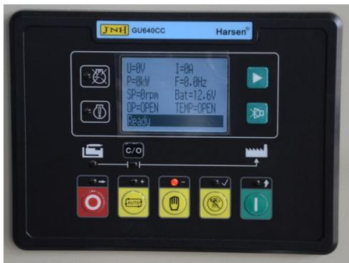
Standard control panel can satisfy the Genset for normal operation, it has the advantages of simple operation, multiple functions, reliable protection. The panel can receive remote open/stop control signal for Genset. (ATS control)
