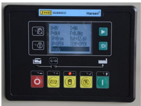
Automatic control panel is the basic configuration of Automatic Gensets of unattended operation. The panel can receive remote open/stop unit control signal. (ATS control)
